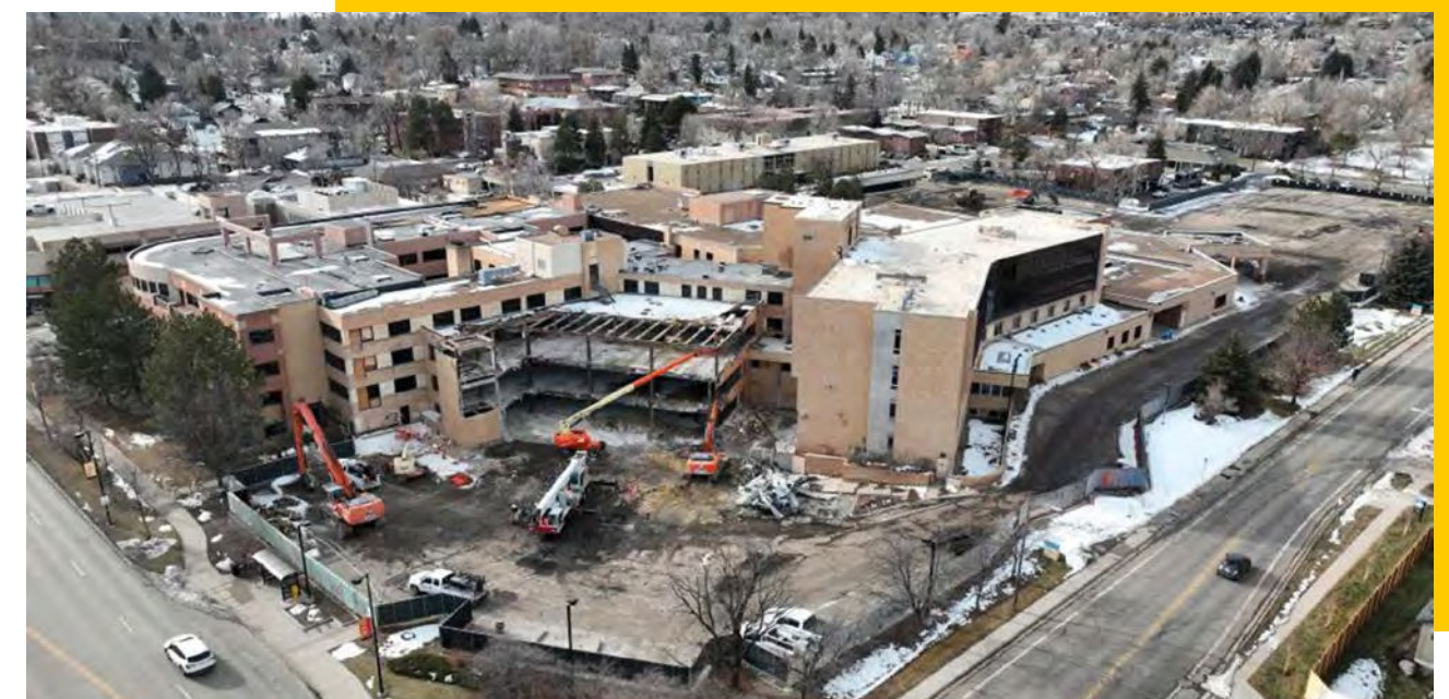
Rückbauarbeiten am Boulder Community Health Hospital | Foto: City of Boulder
